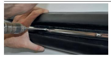
Drill holes in the boat using the same holes of the bars as a guide.
