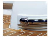
Once finished, finish with silicone on the head of the bar and install the end cap which must partially overcome the end of the profile (it must not be fixed on its side).
